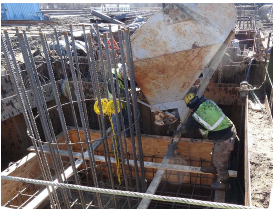
Figure 5.8 US 34 Bridge Pier 2 footing concrete placement
