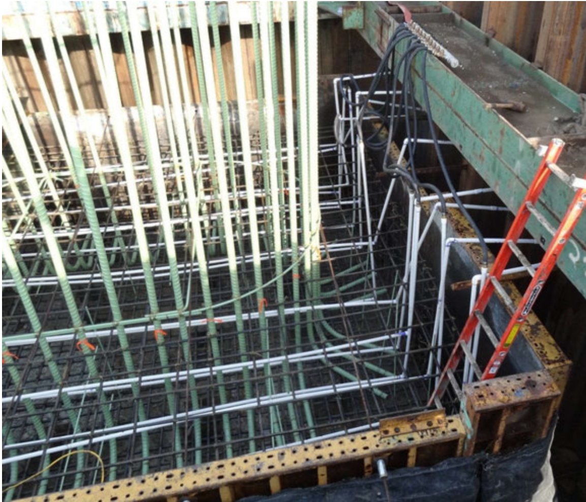
Figure 5.20 Installed PVC piping on US 34 Bridge footing
