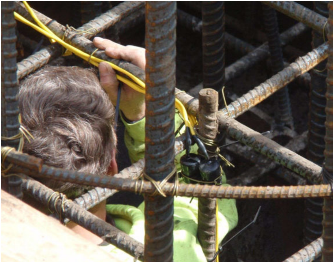
Figure A.1 Installation of thermal sensors with cable ties and tie wire
