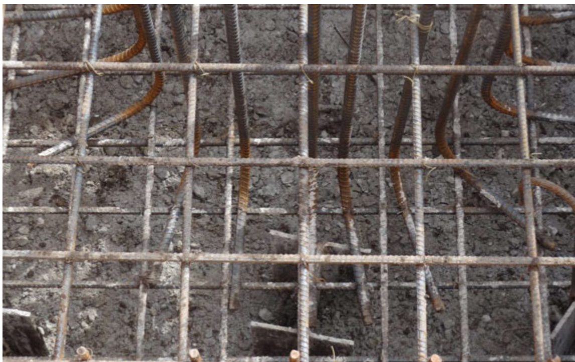
Figure 5.2 Crushed rock subbase with steel bearing pile
