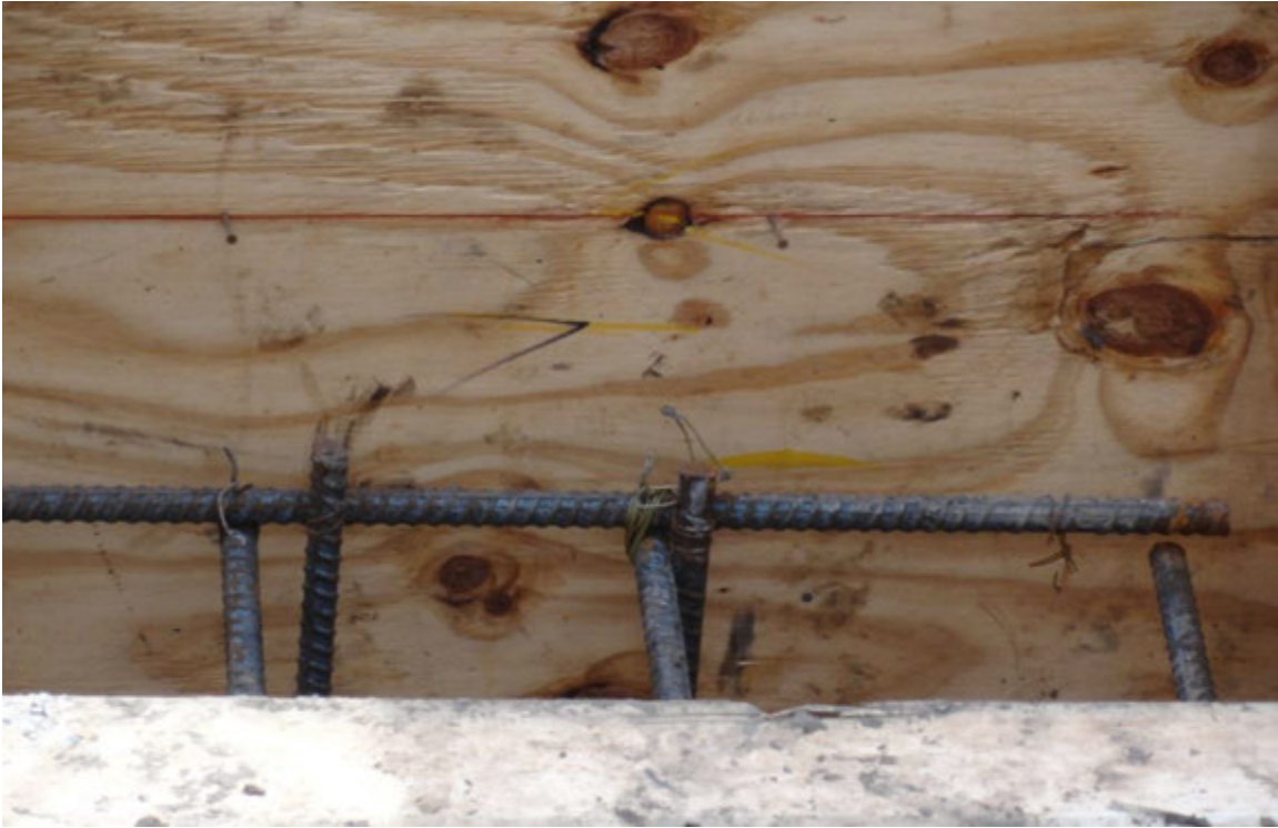
Figure 5.23 Typical rebar cover for mass concrete footing
