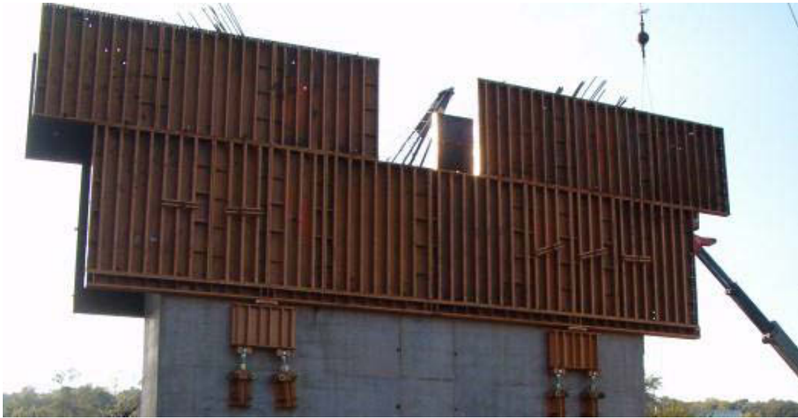
Figure 5.4 WB I-80 over the Missouri River Bridge column formwork
