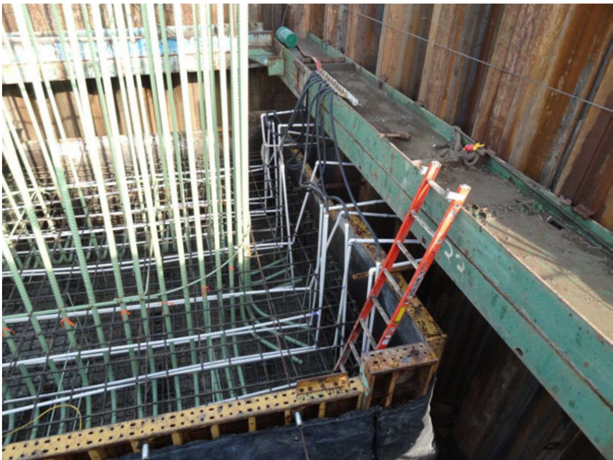
Figure 2.5 PVC post cooling system
