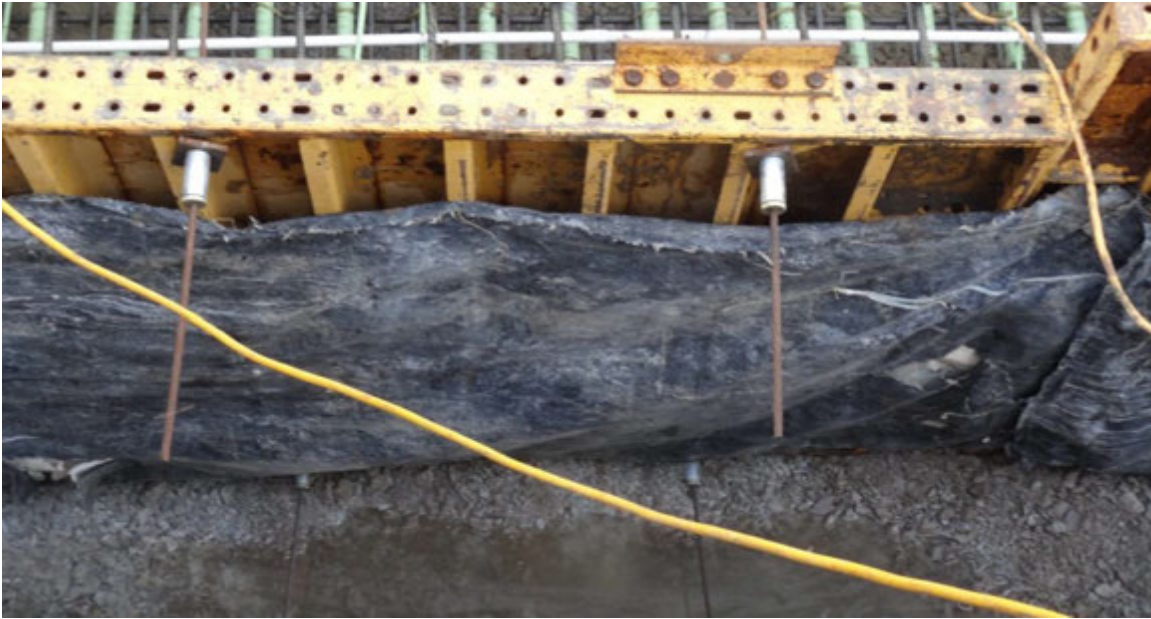
Figure 5.14 Steel formed footing with insulating blanket
