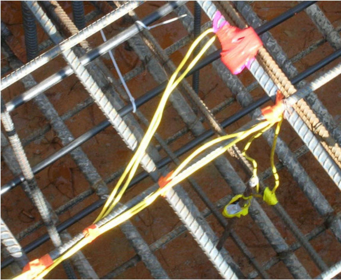
Figure A.2 Top surface and center sensors installed with electrical tape
